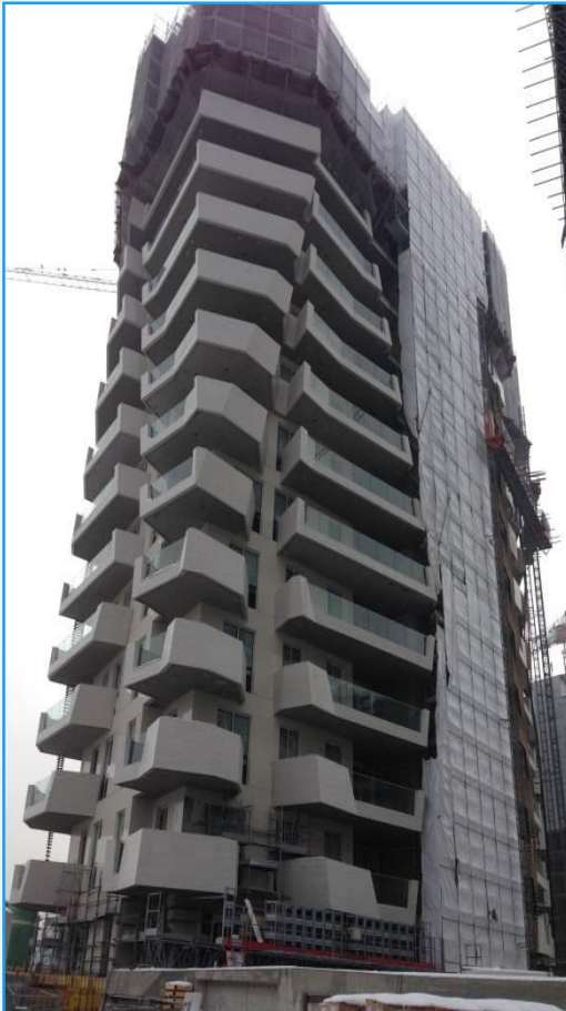
A photograph of a multi-story building under construction, heavily covered in scaffolding. The building has a modern, angular design with white concrete balconies. The construction site is surrounded by other buildings in an urban setting.
